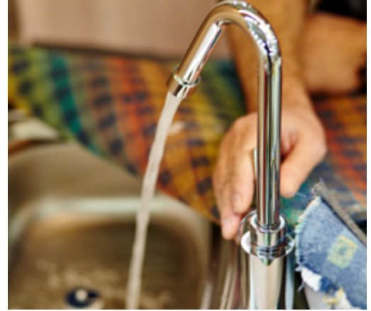
Correct installation of the hydraulic systems.
