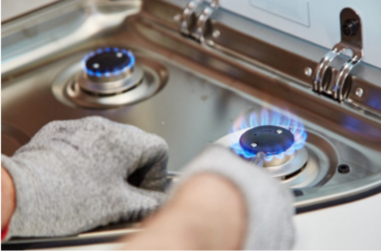
Test on operation of the gas pipes.
