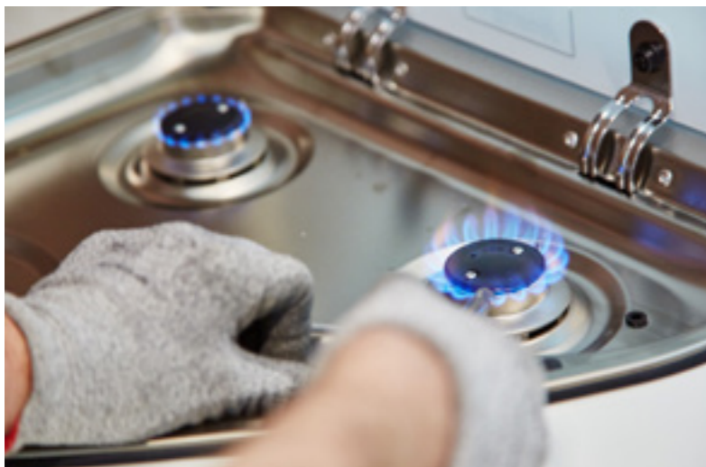
Test on operation of the gas pipes.
