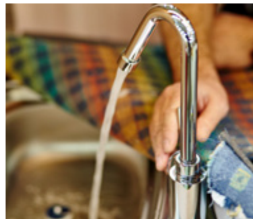
Correct installation of the hydraulic systems.
